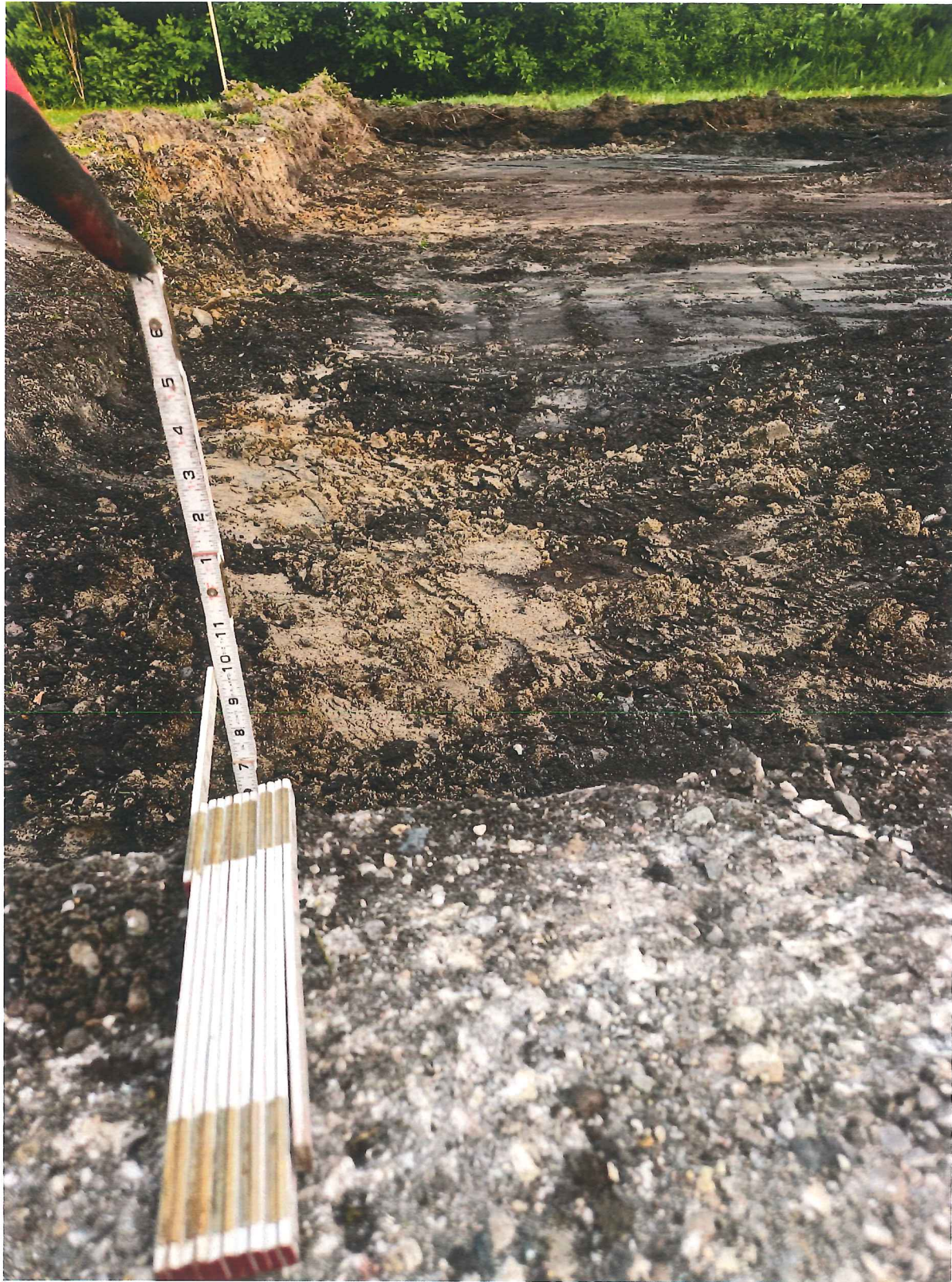
Clinton Valley Elementary Northwest parking lot - existing paving cross section
